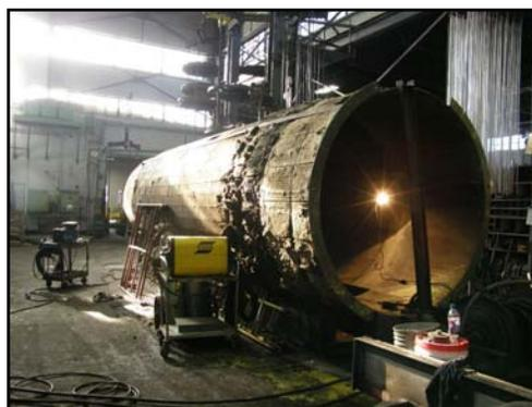
Removing the insulation from the outside of the salt tank.
